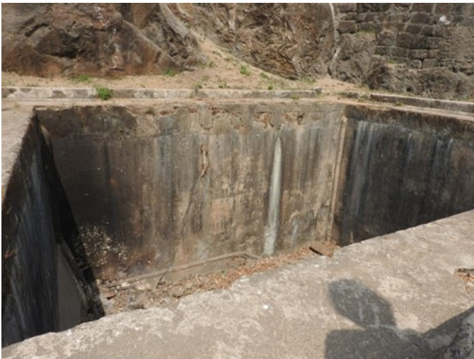
This existing water reservoir, which is currently empty, needs repairs and investigative works to search out the cause of possible leakage or damage, as this once served as a water harvesting system.
