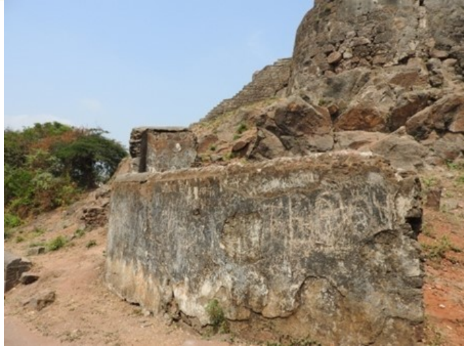
Parapet walls around the fort needs repairs and at some locations they seem unnecessary.
