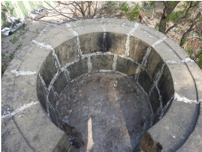
Inappropriate pointing work has been previously done.
