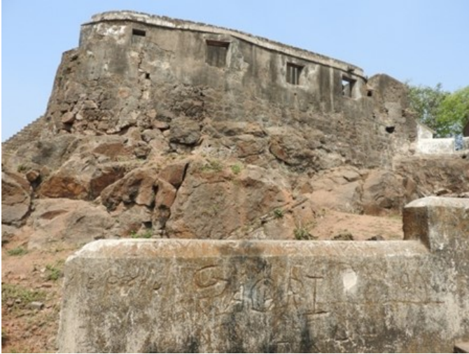
Crumbling stones of the walls need immediate stabilization.
