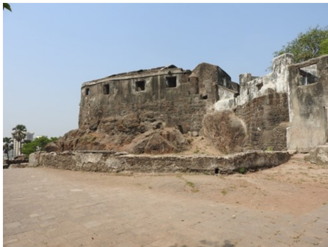
The parapet walls around the open area and landscape need repair work.
