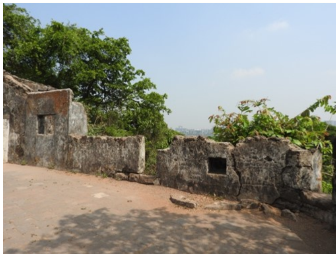
The parapet walls around the open area overlooking the city need repair work.
