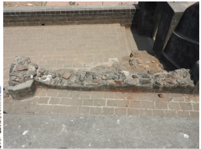
Broken dilapidated walls needs stabilization and consolidation.
