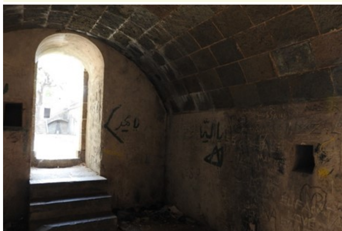
Damaged Walls, Plaster Work and Graffiti.
