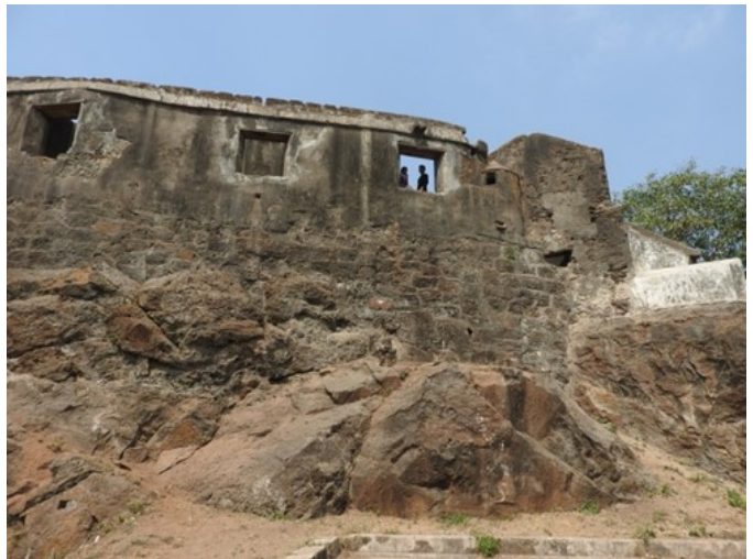
The rocky terrain on which the walls are standing today is still visible. The walls need immediate stabilization and cleaning work, re-plastering work, using traditional and suitable mortar mix.
