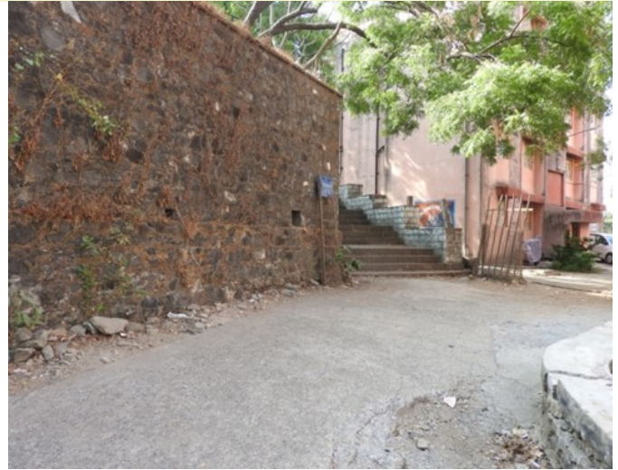
Outer fortification walls of the Fort with missing plinth protection and poor signage.
