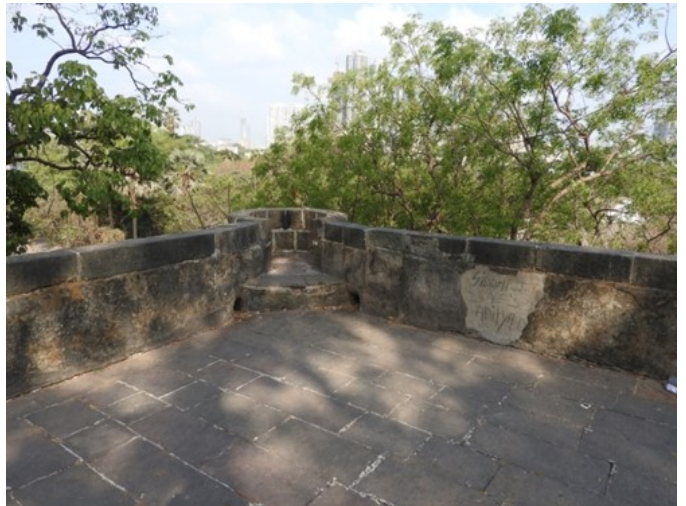
Patchy plaster works should be redone using appropriate method and materials
