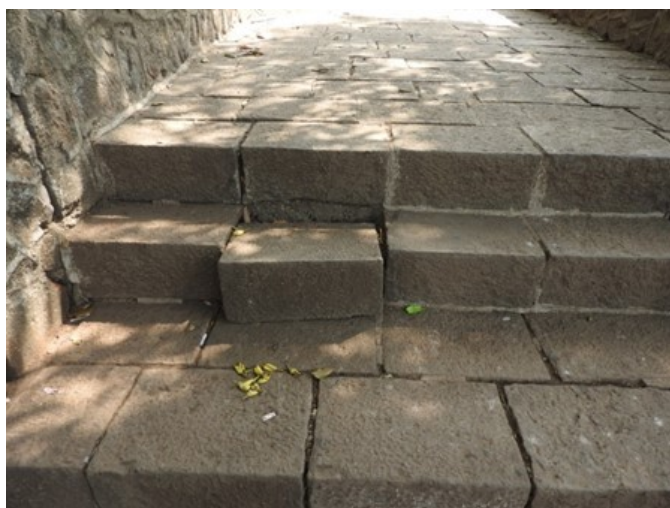
Loose stones in the steps need immediate stabilization.
